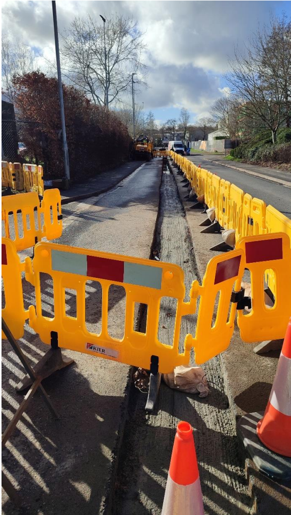
Figure 14 Installation in progress on Osprey Road
