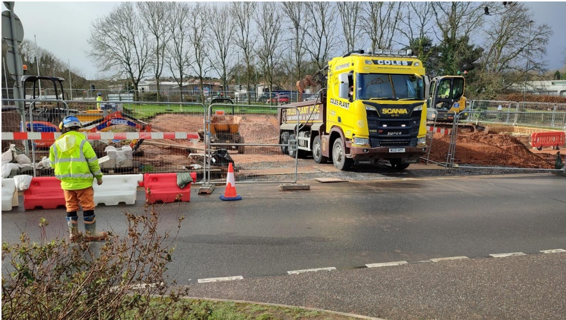
Figure 17 Vehicles removing material from substation site
