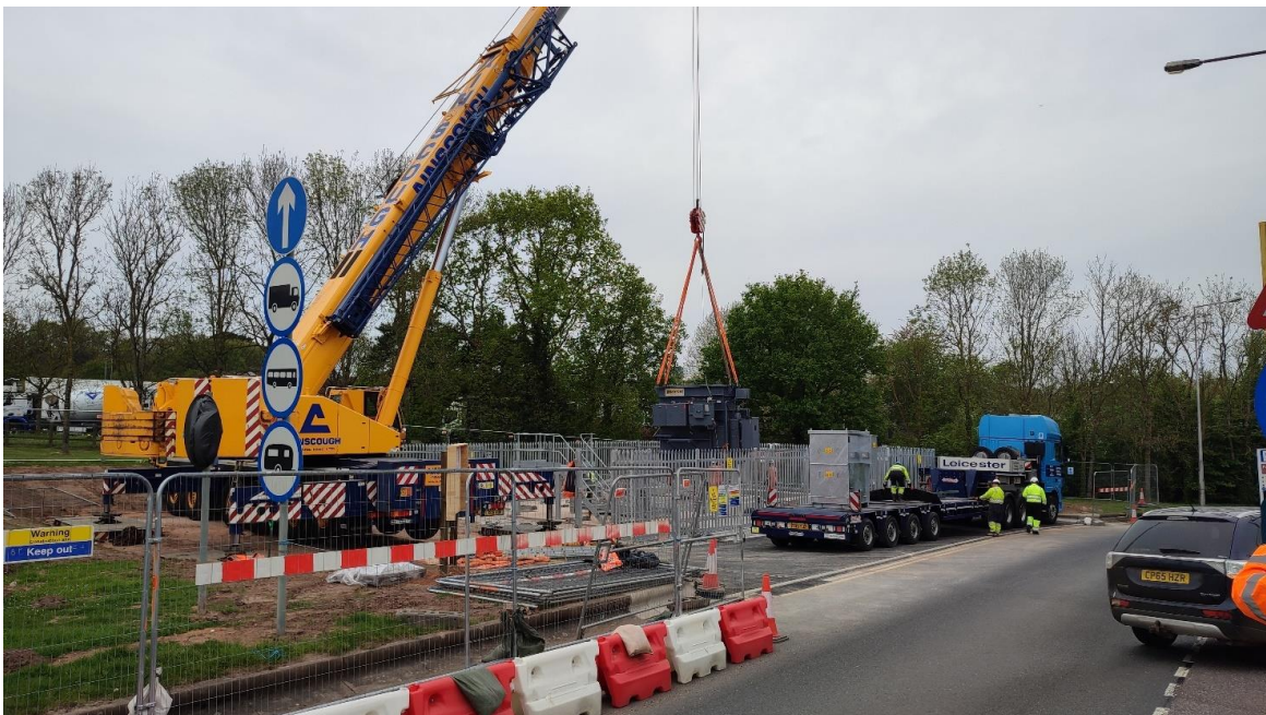
Figure 18 Offloading the 33/11 kV transformer
