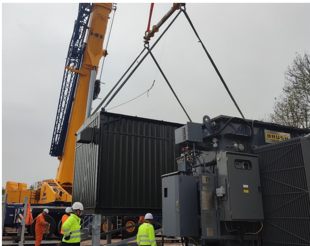
Figure 25 Switchroom container being lifted into place
