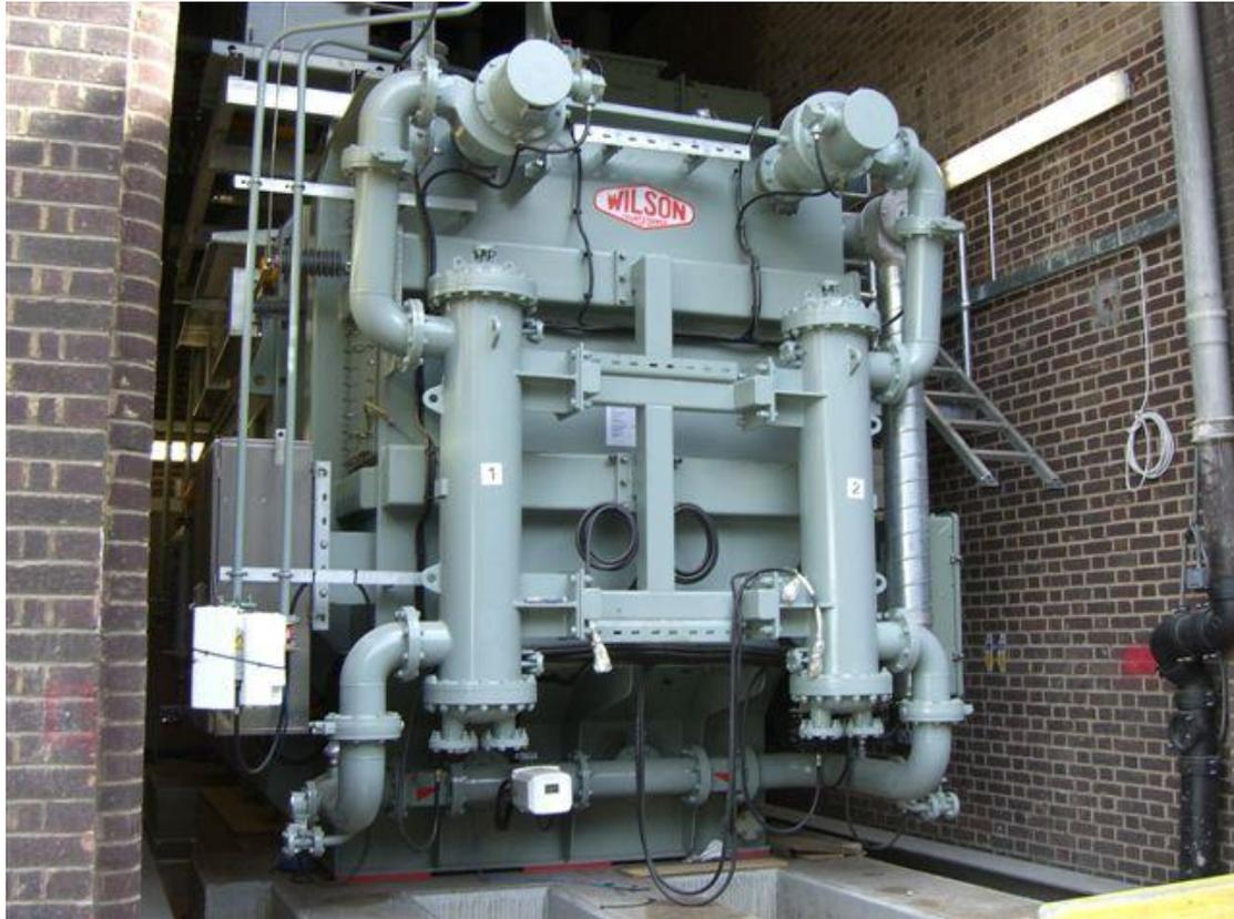
*Figure 24: OFWF transformer at Tate Modern substation*
